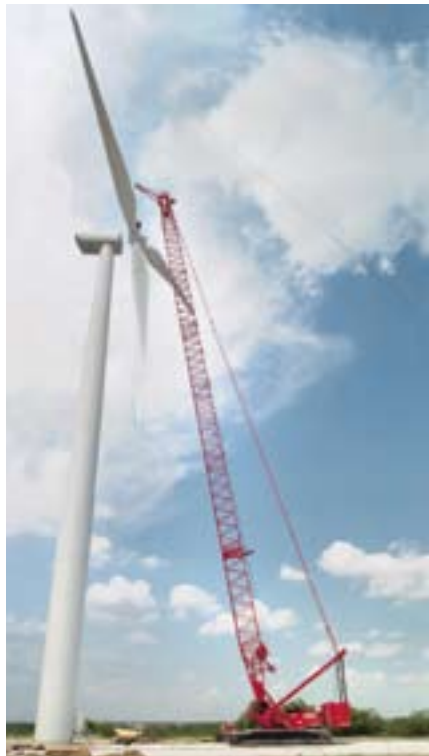
In June 2008, Essex Crane Rental’s Manitowoc 16000 sets the top tower section on a wind turbine project for Milco Constructors
