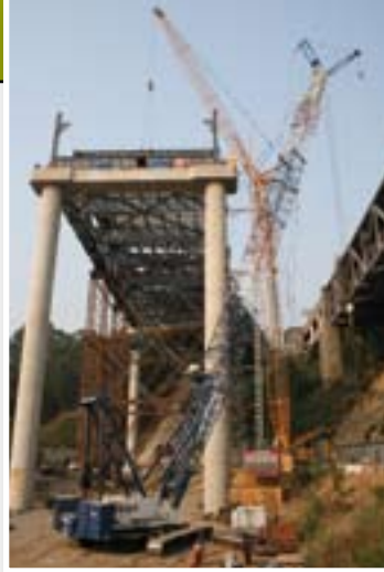
Bigge's Manitowoc 2250 and Liebherr LR 1300 working on the San Francisco Oakland Bay Bridge
