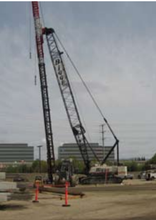
Bigge's American HC 165 driving piles at San Jose International Airport
