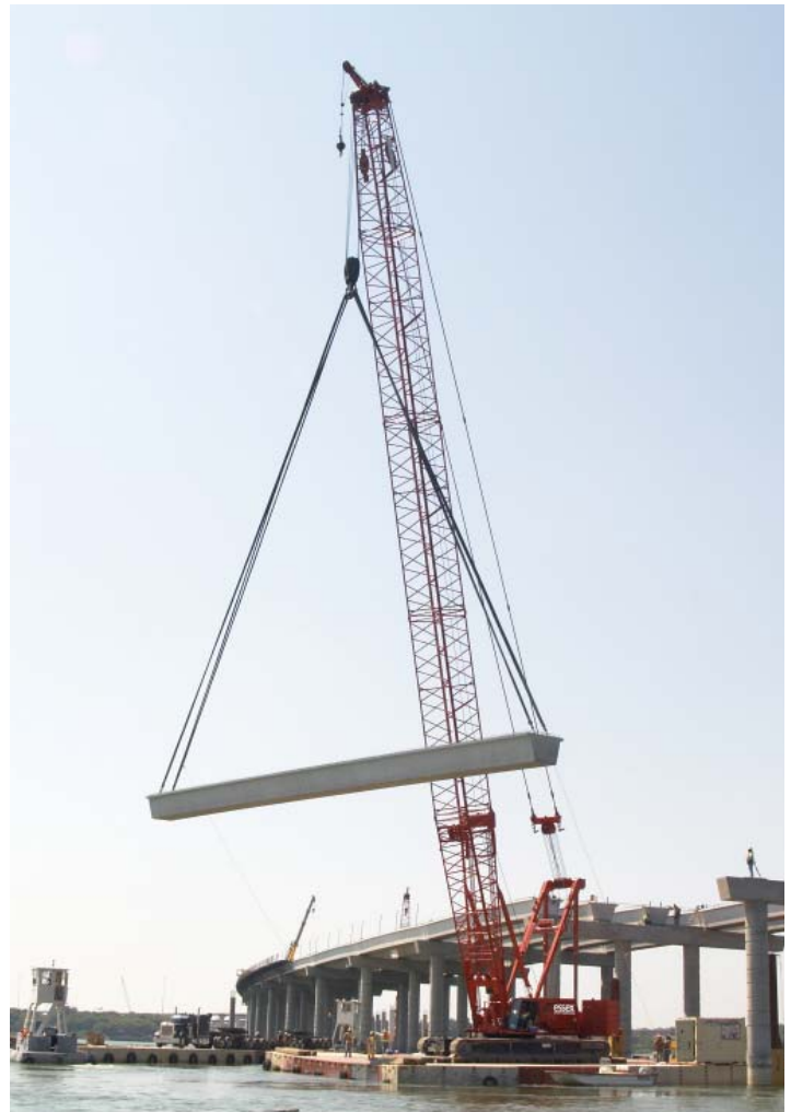
Essex's Manitowoc 2250 SIII lifts 105' long and 142,000 lbs beam at 55' radius
