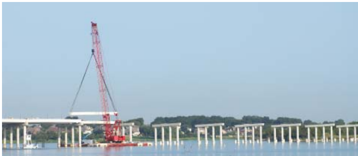
Essex's Manitowoc 2250 SIII lifts 105' long and 142,000 lbs beam at 55' radius
