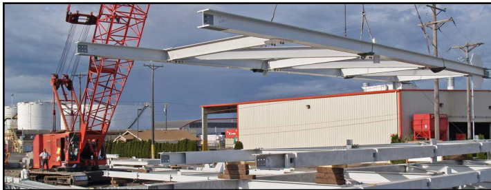
A Manitowoc 4100W from Essex was used to assemble the massive roof trusses at a site across the waterway.
